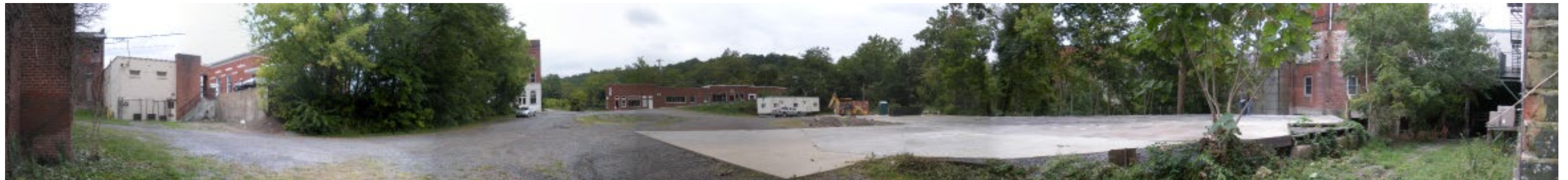
^ view from the NW end of the site towards Church St. before construction.
