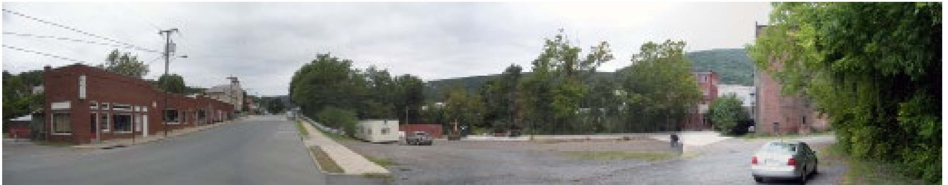
^ overlooking the site (on right) from Church St. (on left) before construction.
